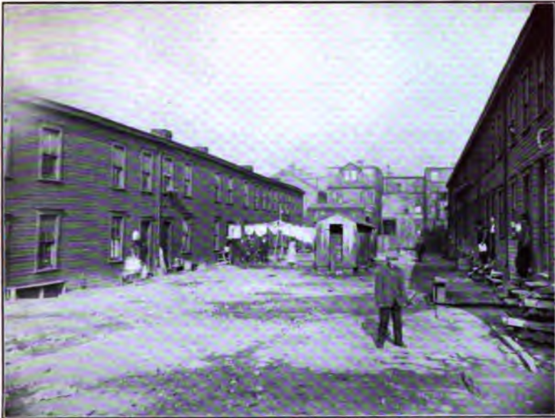
LIVING CONDITIONS, SHARPSBURG Lower Eleventh and Twelfth streets. Central privy vaults used by families in both rows. Two hydrants
